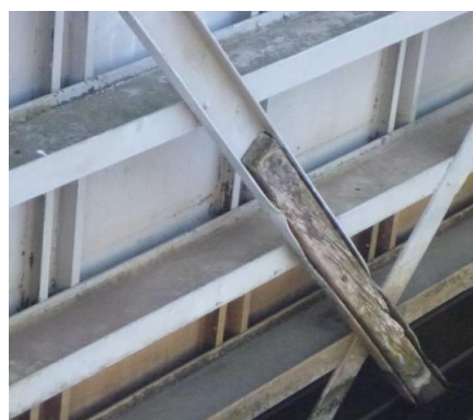
deformace OK vrat DO
